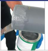
Effast PVCu cement Effast ABS cement Brush (half the diameter of the socket)
